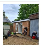
the old ramp has been removed as it was crumbling and didn't meet modern regulations. A new metal ramp, which is fully compliant with accessibility regulations has been fitted in its place.
